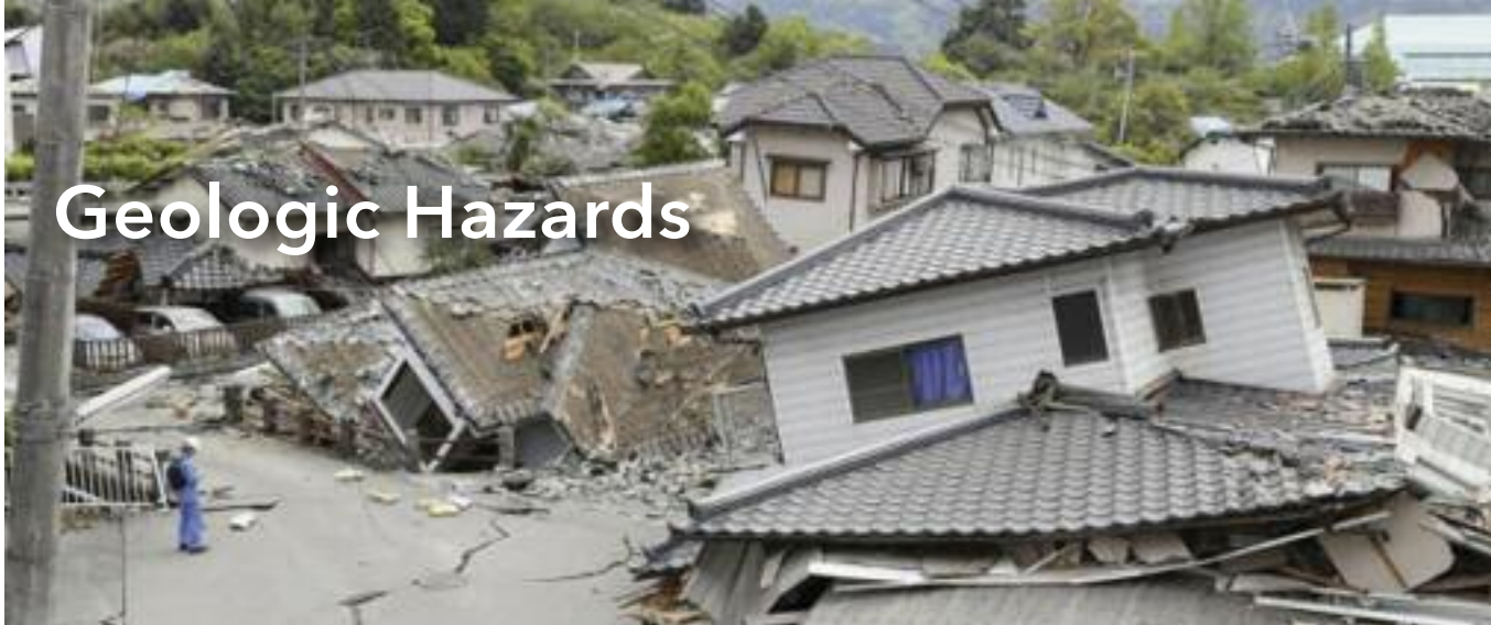
Damaged houses sit after an earthquake in Mashiki, Kumamoto prefecture, southern Japan Saturday, April 16, 2016. Powerful earthquakes a day apart shook southwestern Japan, as thousands of army troops and other rescuers on Saturday rushed to save scores of trapped residents before weather turned bad. Credit: Kyodo News via AP
